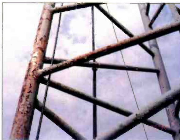
Removing rust to bare metal on a broadcast tower requires an application of a zinc-rich primer. (Photo courtesy of Broadcast Communications, New Glarus, WI.)
